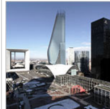
A Defiant Architect's Gentler Side
